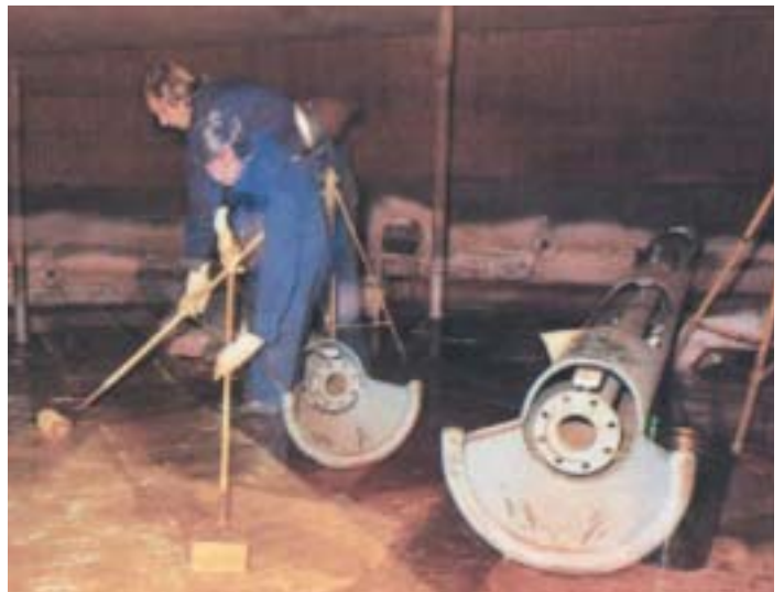
Spreading LEYCO-POX 171S resin binder
