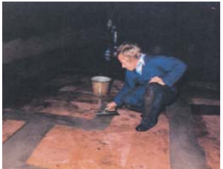
Smoothing irregularities with LEYCO-POX 171S mortar
