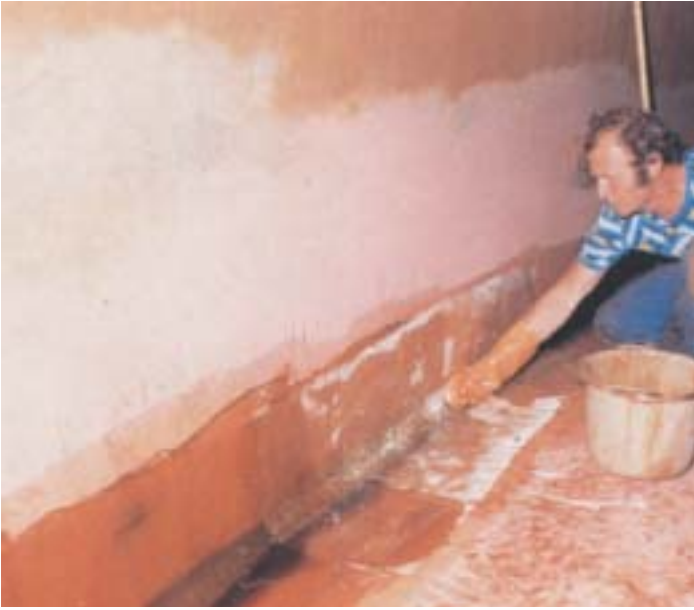
Applying laminate to edge of bottom/wall corner
