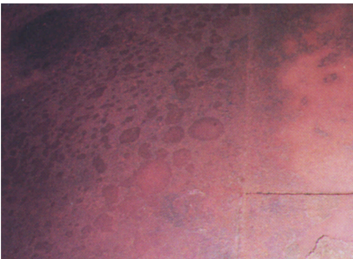
Close-up view of repair of corroded tank bottom
