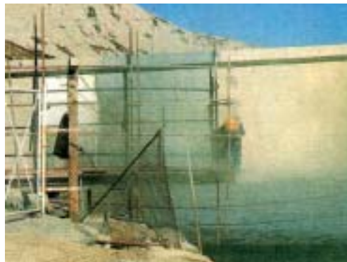
Waterproofing and Protection of a dam
