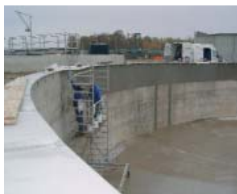
Coating the waterlevel zone of a sewage tank with LEYCO-PLAST AC as protection against corrosion
