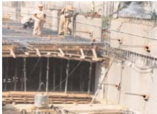
Using of LEYCO-PLAST AC during tunnel constructions for waterproofing
